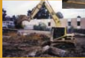
Building of new facilities at 917 Main Road, Eltham, 1995.
